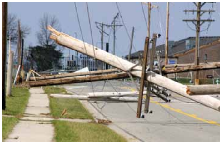
Keep family and friends away from all downed power lines.
