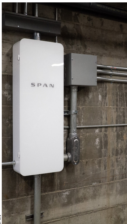
With smart breaker boxes, like the SPAN Panel shown here, you can control and monitor every circuit in your home from a smartphone or tablet.
