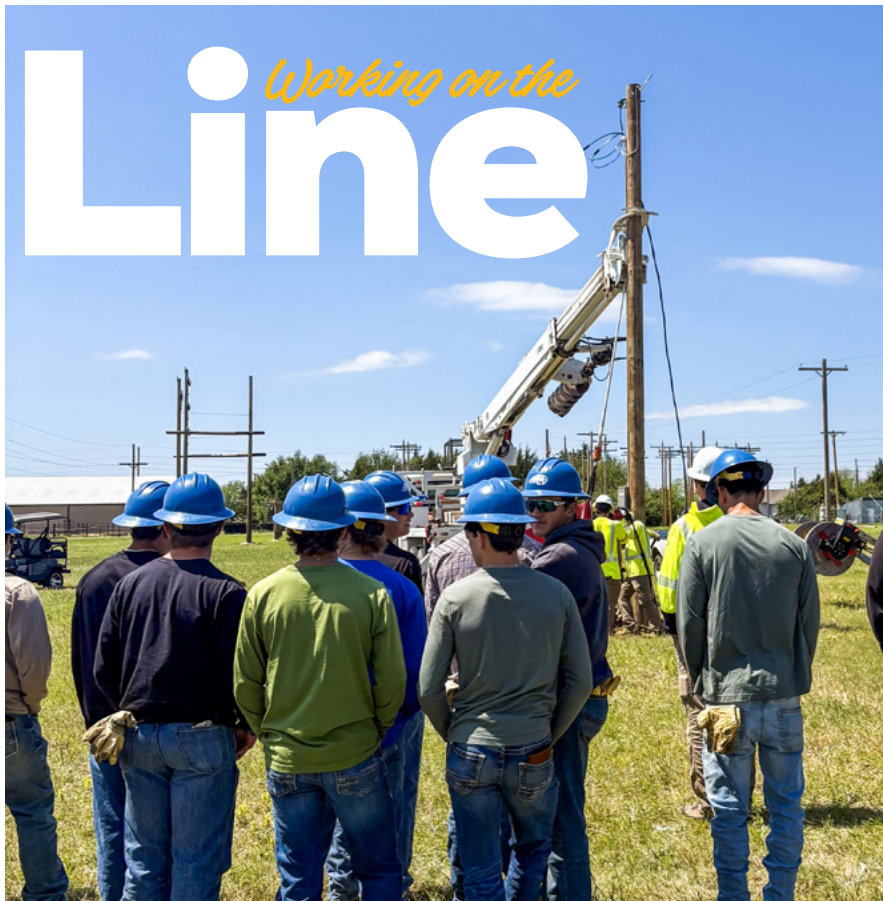
Ninnescah linemen demonstrating a mock construction build for Pratt Community College's Electrical Powerline Technology students.
